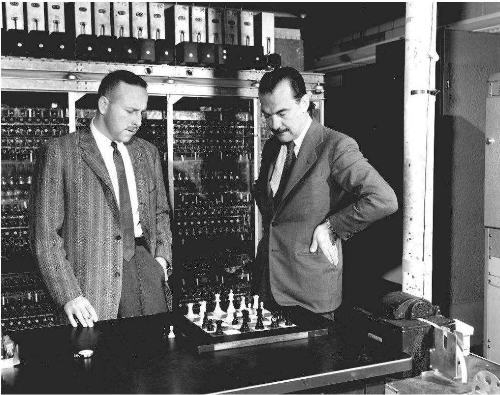
Fig. 2. One of the early computer chess programs was written for the MANIC computer built at Los Alamos Scientific Laboratory. The computer's paper tape reader/puncher was used to communicate all the chess moves. Source: www.armageddonchess.webs.com
